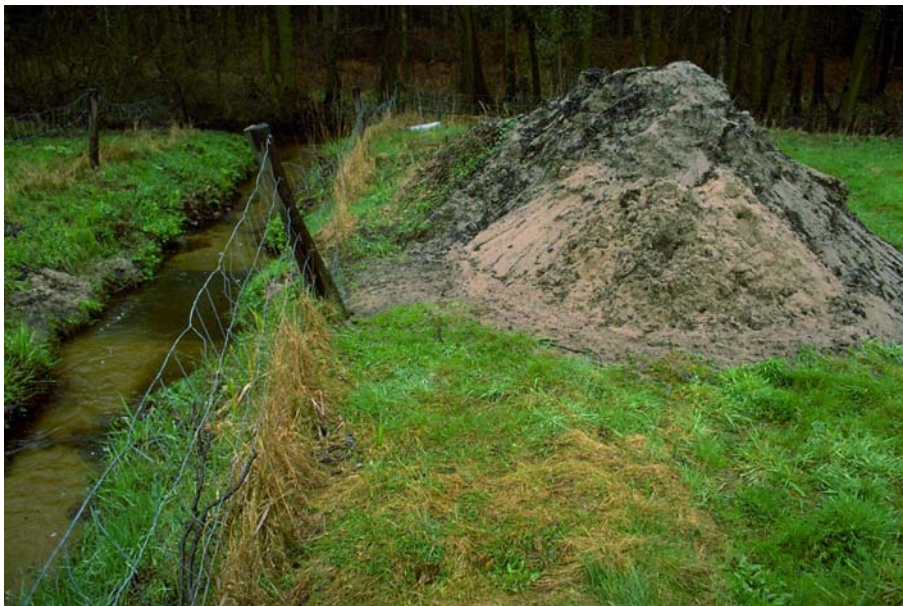
Fig. 2: Sediment trap in the Endeholz Ditch just before the confluence with the Lutter river (background) with the mound of sandy and organic material which was taken out of the trap from 1991 to 03. April 1998. The size of the mound shows the large amount of material carried by this small ditch.
